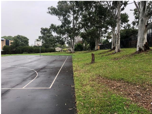
Figure 28: View west along north boundary of study area showing courts and excavated slope.
