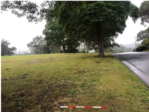
Figure 34: Slumping at location of the former Kishnaghur
