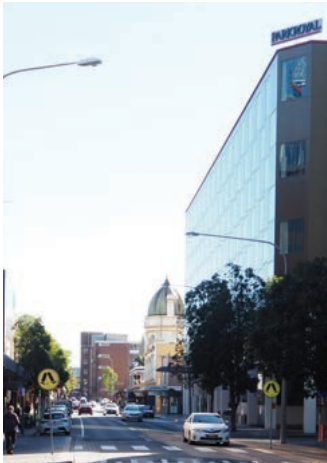
Figure 15: View looking west down Phillip Street towards to the former ANZ bank building. Note the sympathetic street frontage setback for the adjacent buildings to the east retain clear views of the historic building.
