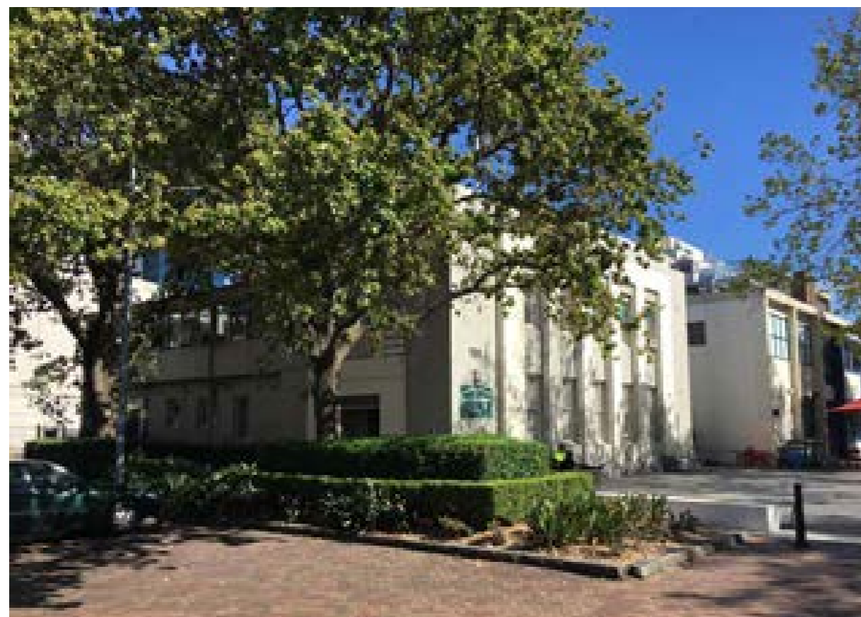
St John's building from Cathedral carpark
