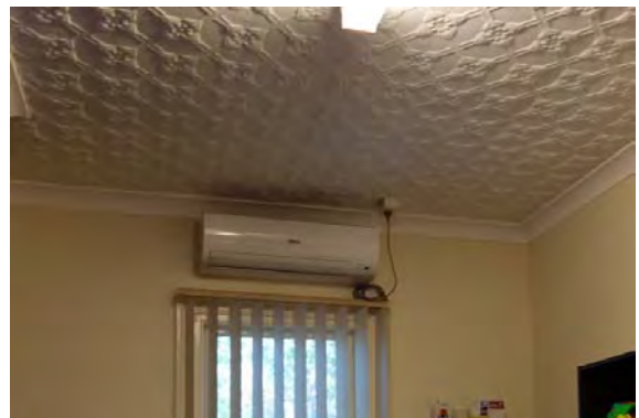
Figure 2.3.61: Section of extent pressed metal ceiling within one of the main rooms of the former cottage.
