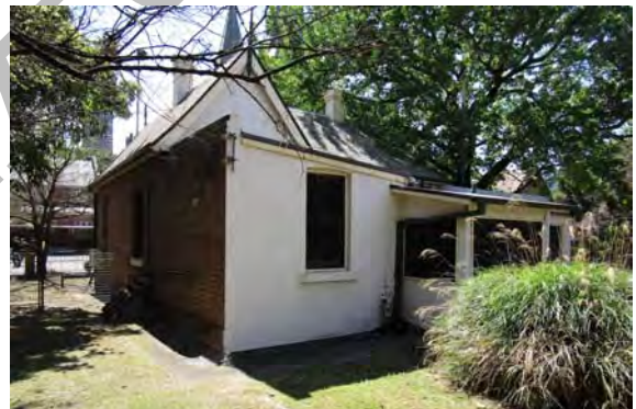
Figure 2.3.59: Rear and side (west) elevations of the former Verger's cottage.
