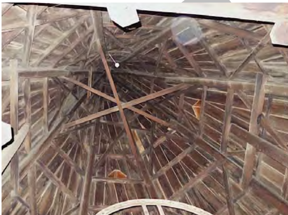
Figure 2.3.42: Timber framing and boarding of the copper clad spires (North tower).
