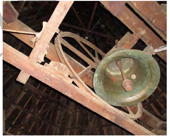
Figure 2.3.50: Timber pulley and 1866 bell within the North tower.
