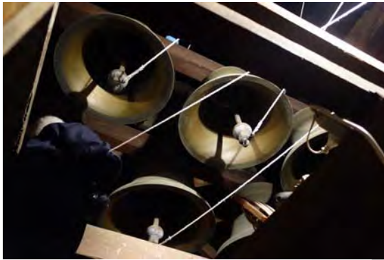
Figure 2.3.53: Carillon of 13 bells dating from 1923 located on Level 3, South tower.
