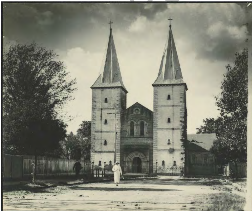
Figure 2.1.27: Photo of the western façade and towers c1920 showing the iron fence and gates at the end of Hunter Street (Source: SLNSW)
