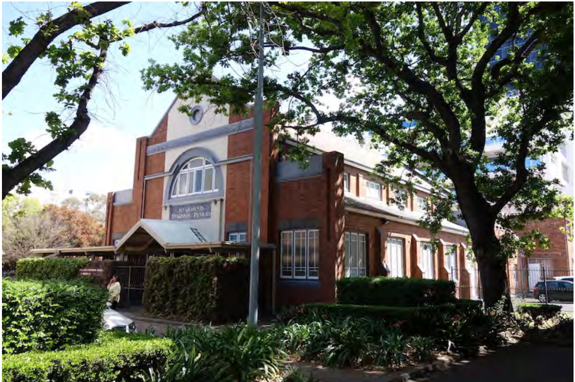
Figure 2.3.64: St John's Parish Hall.
