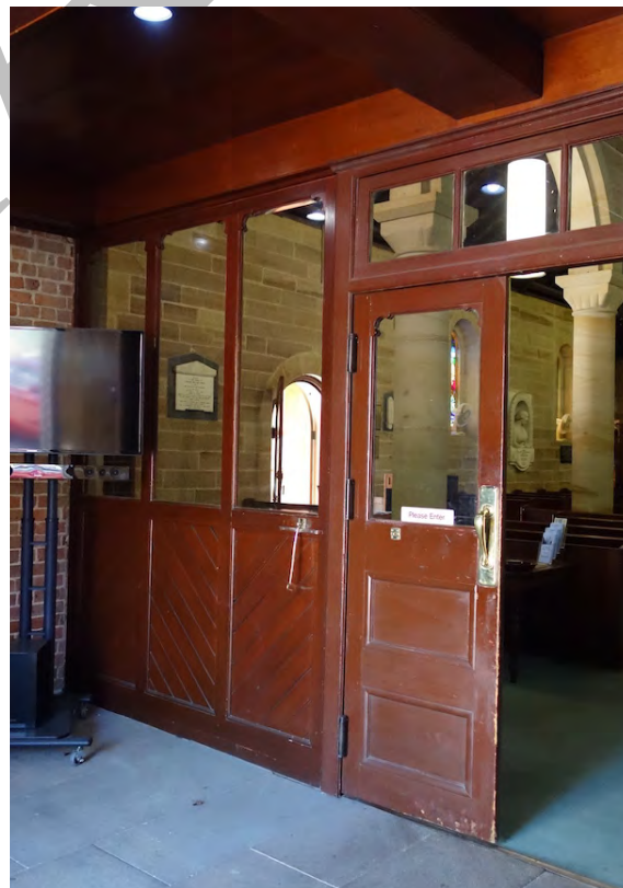
Figure 2.3.33: 1960s timber screen between the western entrance and the nave.
