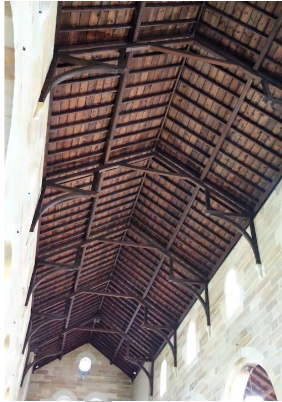
Figure 2.3.31: Hammerbeam trusses and timber boarded ceiling over the nave.
