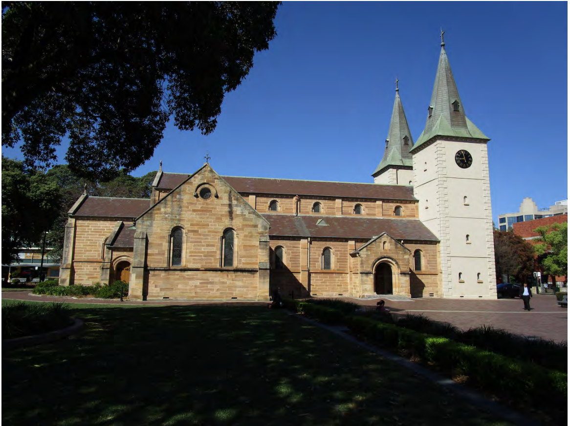
Figure 2.3.16: St John's Cathedral facing Centenary Square (north elevation).
