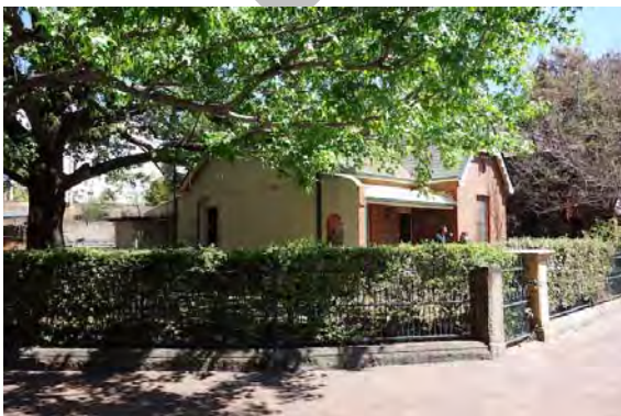
Figure 2.3.60: Former verger's cottage from the east, bound by modern steel palisade fence.
