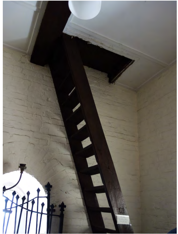
Figure 2.3.48: Steep stair access within the North Tower between Levels 1 and 2.
