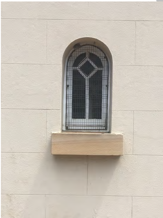
Figure 2.3.20: Typical ground level window to the towers.
