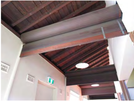
Figure 2.3.71: Original roller shutters separating the side aisles in to smaller classroom spaces.
