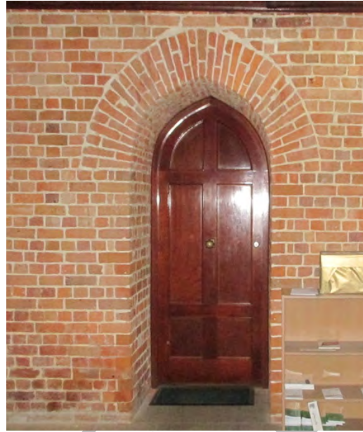
Figure 2.3.35: 1960's timber door to the North tower. Note unpainted sandstock brick.
