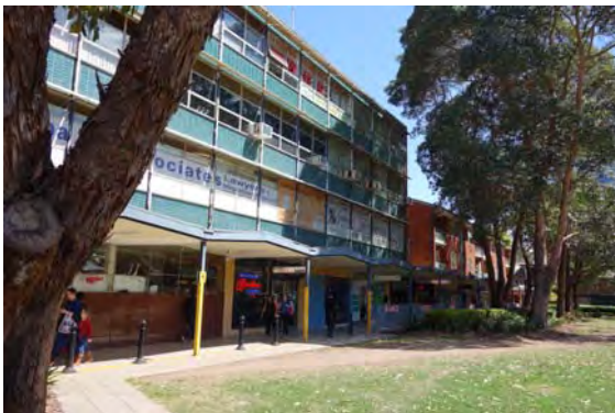
Figure 2.3.7: Queensland Insurance building located to the south of St John's.
