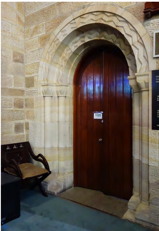
Figure 2.3.32: Typical framed, ledged and braced doors to the former entrance porch adjacent the chancel. Note typical Romanesque detailing of scalloped capital, half-shafts and chevron detailing and framed, ledged and braced door.
