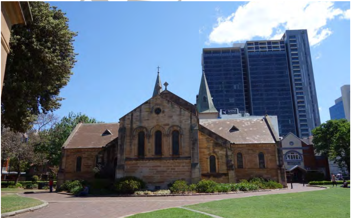
Figure 2.3.17: Eastern elevation of St John's Cathedral facing Church Street.
