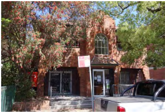
Figure 2.3.77: Former Interwar apartment building at 45 Hunter Street, presently used as the offices for the Anglican Home Mission Society.
