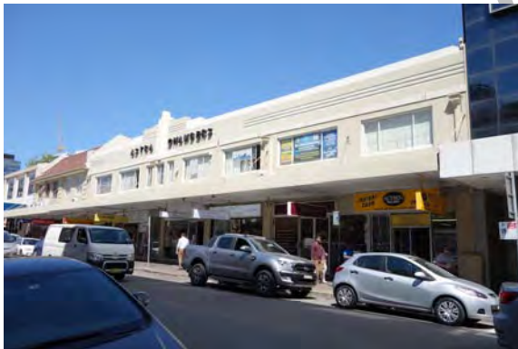
Figure 2.3.81: Commercial building 'Astra Chambers' at 65-73 Macquarie Street
