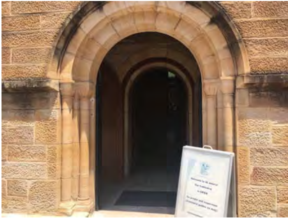
Figure 2.3.22: Northern entrance fronting St John's Square.
