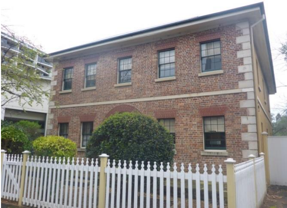
THE COLONIAL HOUSE KNOWN AS HARRISFORD
