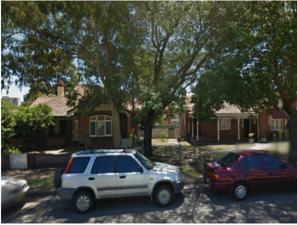
CONTRIBUTORY DWELLINGS FRONTING WESTON STREET
