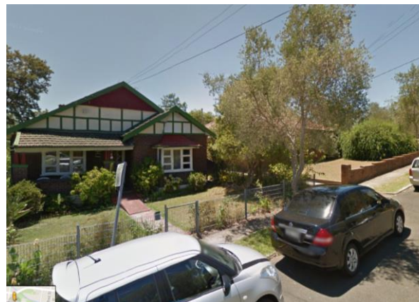
CHARACTERISTIC BUNGALOW DWELLING ON THE NORTHERN SIDE OF RUSE STREET WEST OF THE EXPERIMENT FARM COTTAGE
