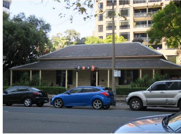
'PERTH HOUSE' 85 GEORGE STREET
