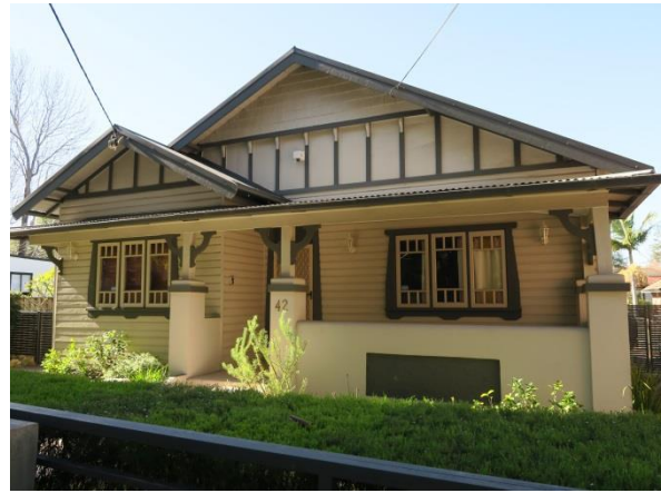
SAMPLE OF INTER-WAR HOUSING STOCK IN THE HCA (THE HERITAGE LISTED DWELLING AT 42 SORRELL STREET).
