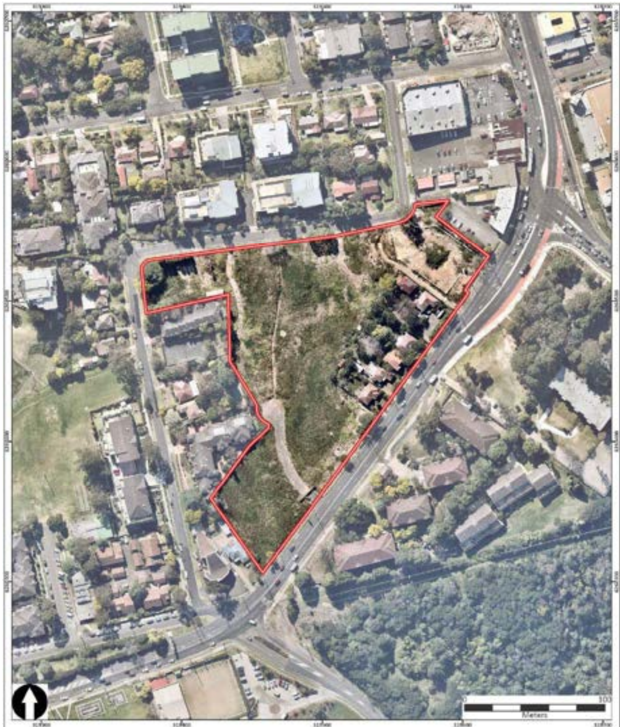
Figure 28. 2017 aerial showing the progressive demolition of Postwar residences on the site. Source: Nearmap with Extent Heritage overlay.
