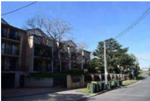
Figure 36. View of the four storey apartment to the west of the site along Shirley Street.
