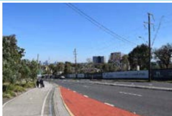
Figure 51. View of the descending topography along Pennant Hills Road.
