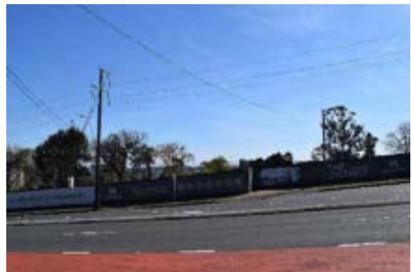
Figure 39. View northwest to the site from Pennant Hills Road.
