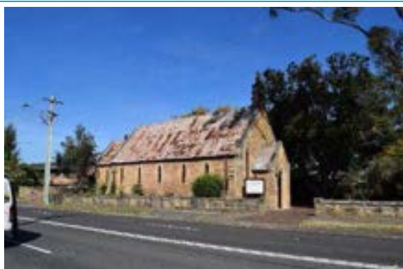
Figure 52. Photograph of the St Paul's Anglican Church (SHR #00056 and LEP I30).
