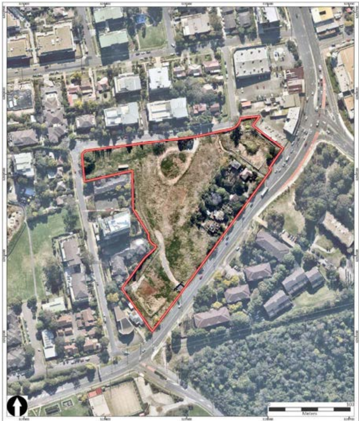
Figure 32. 2021 aerial showing the progressive demolition of Postwar residences on the site. Source: Nearmap with Extent Heritage overlay.
