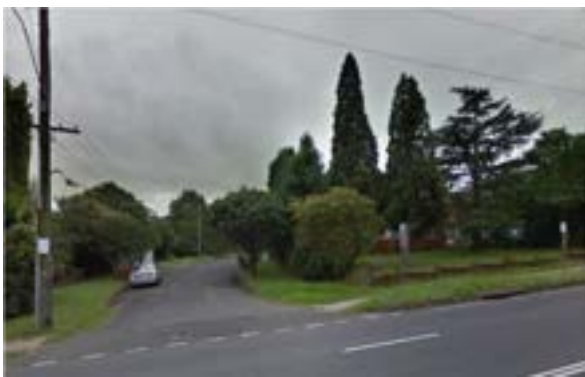
Figure 22. View to Janelle Crescent from Pennant Hills Road prior to demolition. Source: Google Streetview, March 2014.
