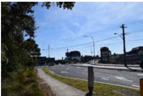
Figure 46. View to the high point of the landscape and commercial buildings along Pennant Hills Road and Marsden Road.
