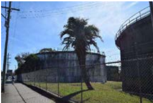
Figure 56. Photograph of the Water tanks and Water Board cottage (LEP I27).
