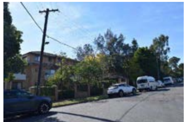
Figure 41. View of the four storey apartment developments along Shirley Street.
