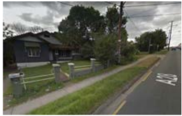
Figure 21. View to the site along Pennant Hills Road prior to demolition. Source: Google Streetview, July 2013
