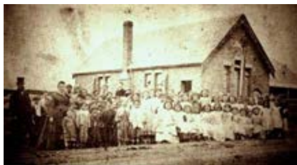
Figure 8. Early photograph of the school hall at the St Pauls Anglican Church. c.1870s. Source: Hornsby Shire Recollects.
