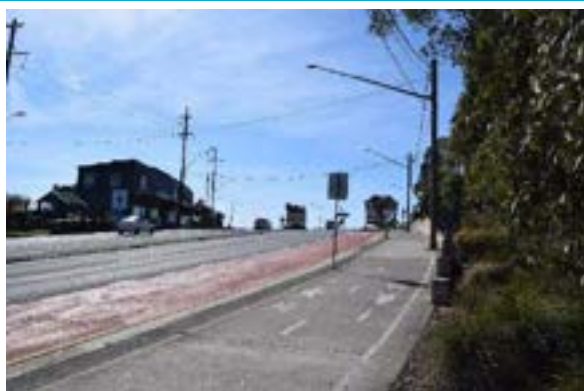
Figure 50. View of the ascending topography along Pennant Hills Road.
