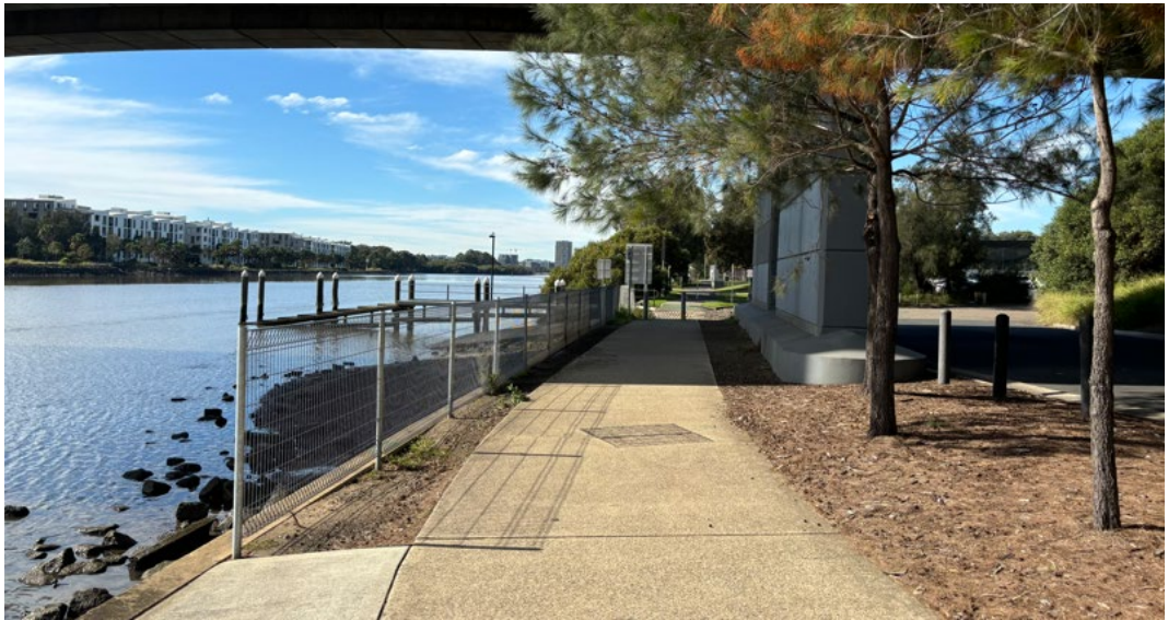
Figure 5 Photograph of an existing footpath beneath Silverwater Bridge
