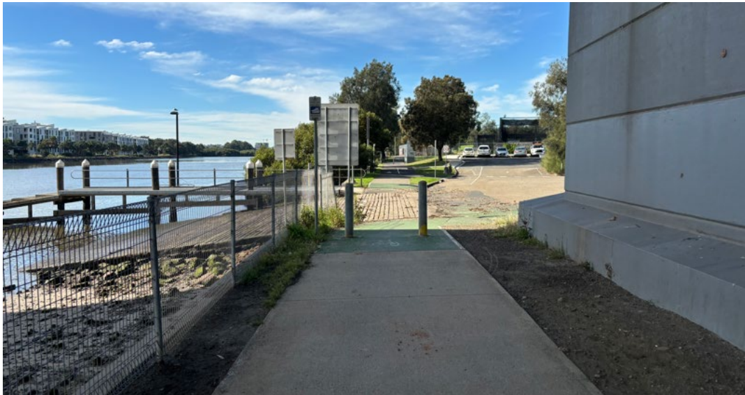
Figure 6 Photograph of an existing boat ramp
