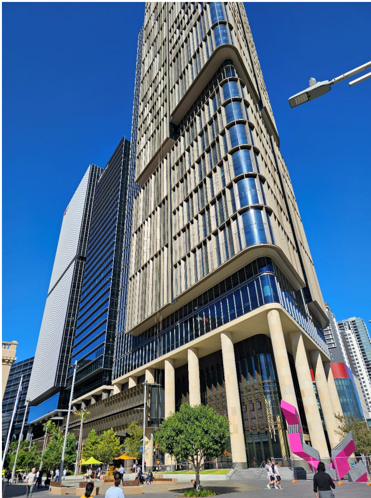
Figure 2 – Recently completed commercial office towers on Walker Corporation Landholdings at Parramatta Square, which is subject to rezoning under this planning proposal (known as 4 & 6 & 8 Parramatta Square).
