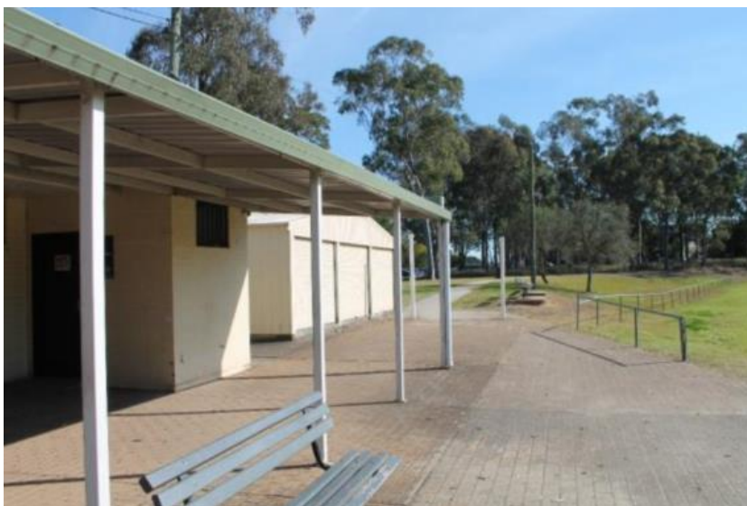
Photograph 2: Existing Amenities Building
