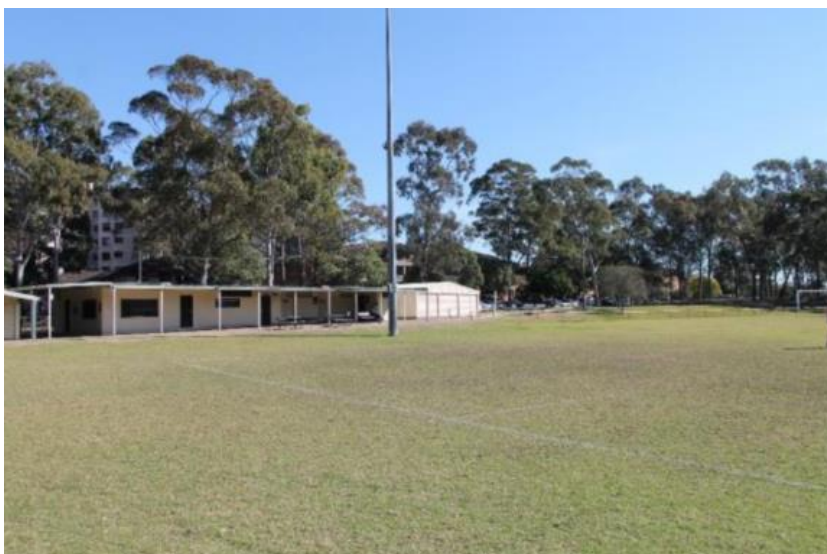
Photograph 1: Existing Amenities Building and Shed viewed from the oval
