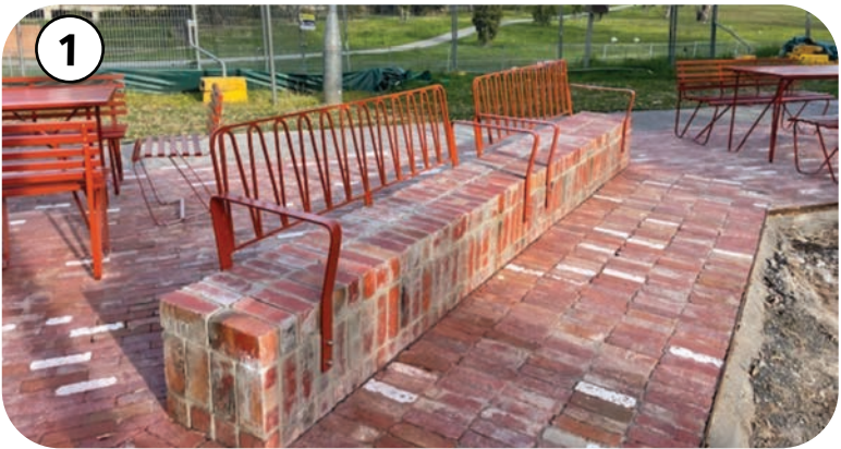
Plate 1-1: Brick Seating Walls
