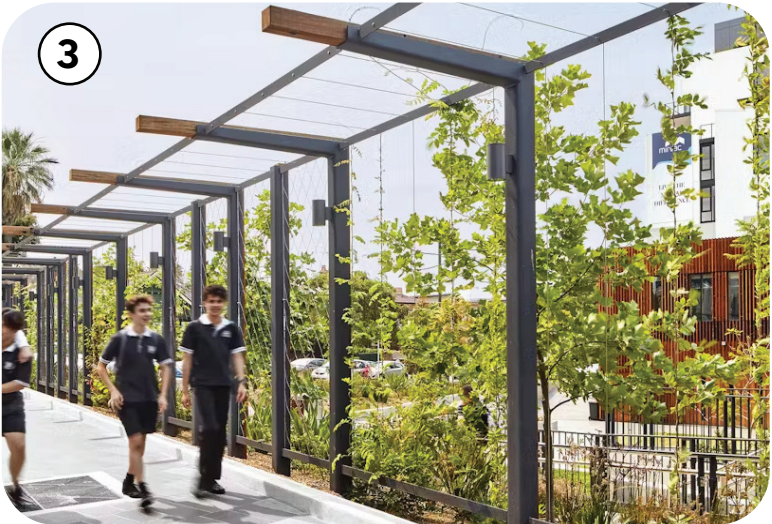
Plate 1-2: Pergola Structure with Lighting
