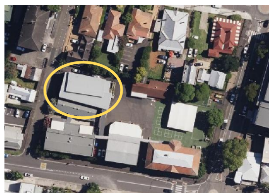
Figure 10. Current aerial, location of former 2 Trott Street dwelling circled in yellow.
