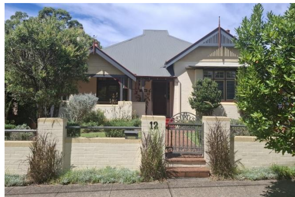
Figure 58. 12 Victoria Street (currently graded as contributory).
