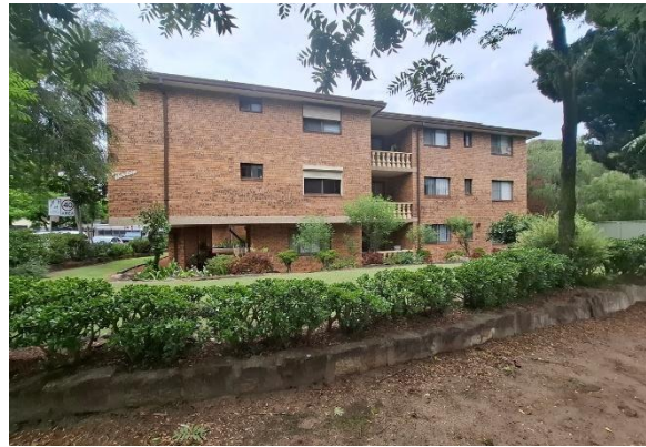
Figure 4. Low rise apartment building at 13 Trott Street (currently ungraded).
