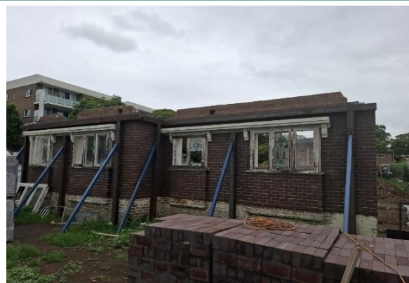
Figure 43. 71 Alice St – contributory dwelling currently being redeveloped.
