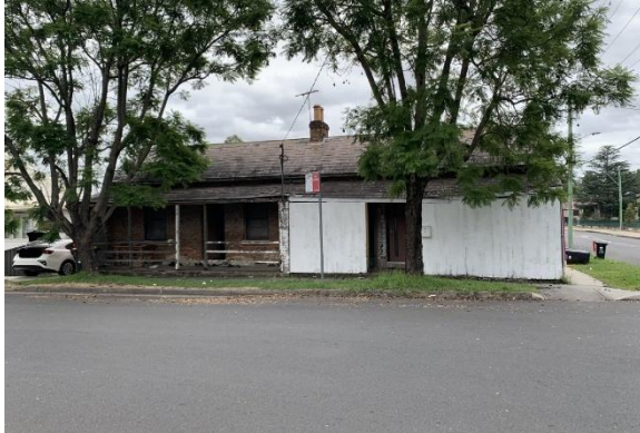
Figure 83. 1-3 Lennox Street which are listed as a pair of cottages.
