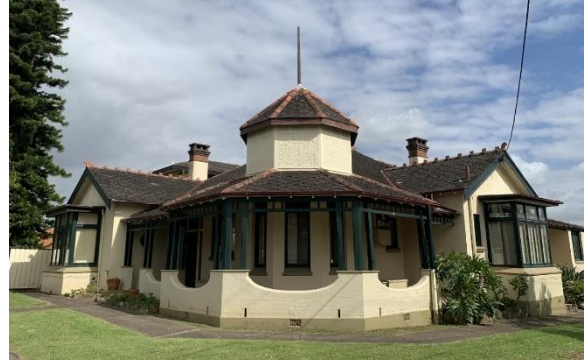
Figure 33. Existing heritage item at 22 Crown Street (I250).
