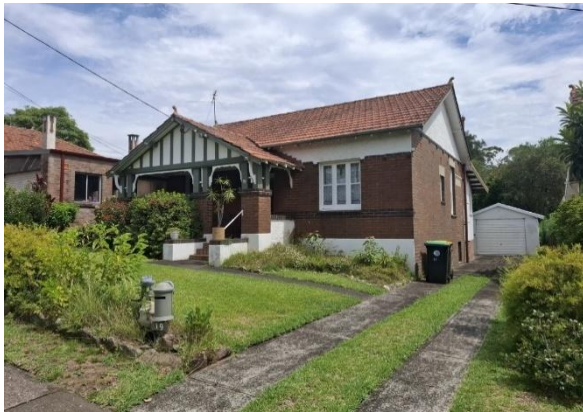
Figure 71. 19 Wyralla Avenue (currently contributory).
