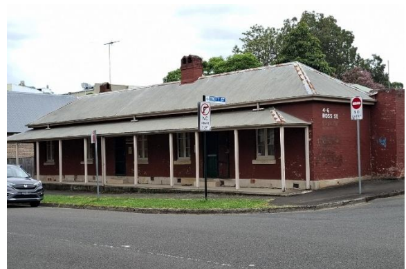
Figure 2. Existing heritage item at 4-6 Ross Street.
