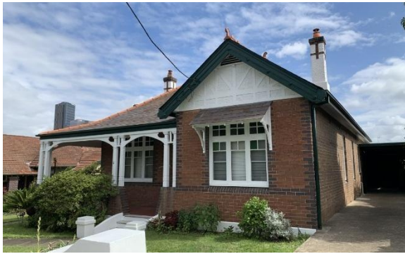
Figure 32. Existing heritage item at 6 Crown Street (I244).
