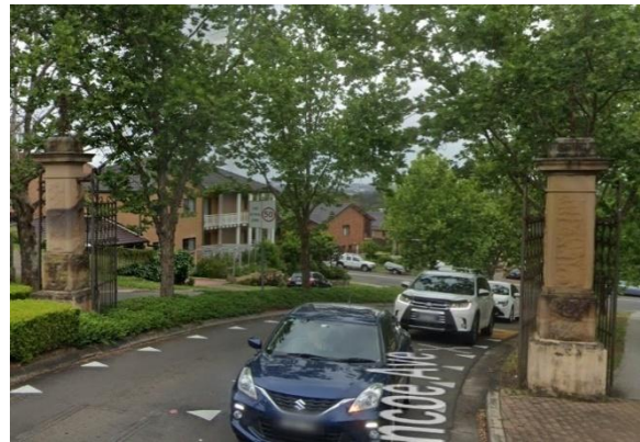
Figure 53. Sandstone gateposts and metal gates – not currently within HCA boundary.
