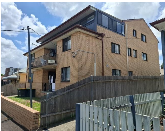
Figure 24. 34 Albion Street (currently graded as contributory).
