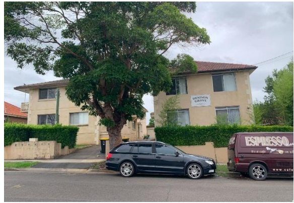
Figure 88. Residential flat buildings at 12-14 Denison Street (currently ungraded).
