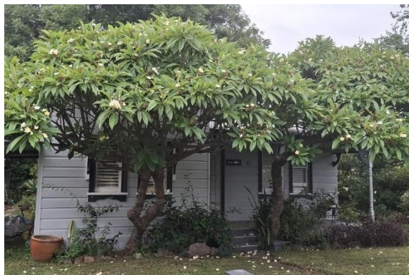
Figure 44. 89 Hassall Street (currently not graded).
