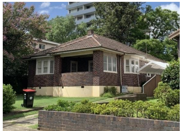
Figure 35. 21 Ruse Street (currently identified as contributory).
