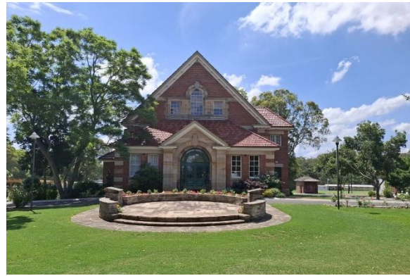
Figure 51. Sargood Hall, 2 Masons Drive.
