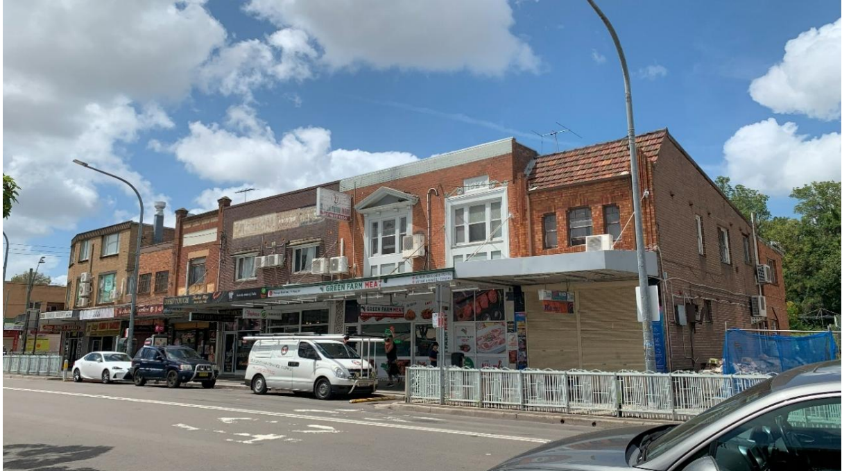
Figure 101. Properties at 55A-59B Marion Street, 60 Wigram Street recommended for inclusion in the Harris Park West HCA boundary.
