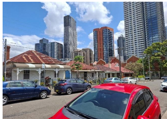
Figure 23. Heritage listed dwellings along Harris Street.
