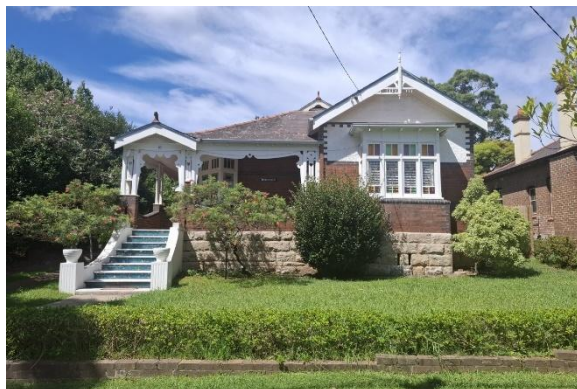
Figure 57. 16 Victoria Street (currently graded as contributory).
