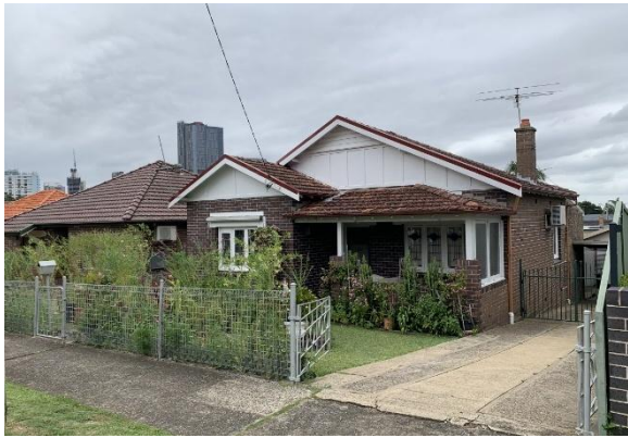
Figure 87. 15 Denison Street (currently ungraded)
