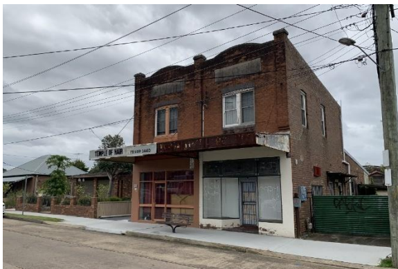
Figure 85. Former terrace shops at 8 Crimea Street (currently ungraded)
