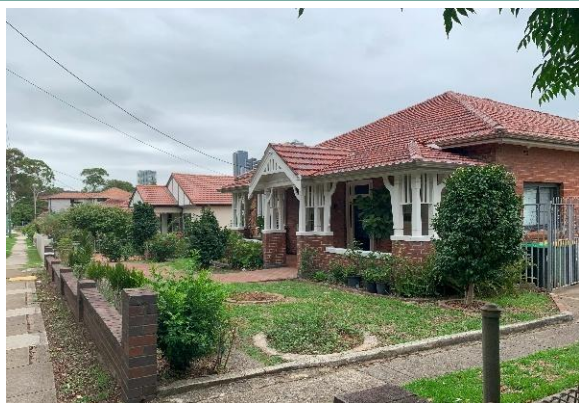
Figure 42. Dwelling at 41 Prospect Street (currently graded as contributory).
