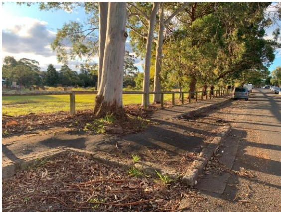
Figure 28. View to stone kerbs and gutters along Short Street.
