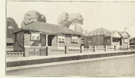
COTTAGES ADJOINING ROSEGROVE ESTATE
