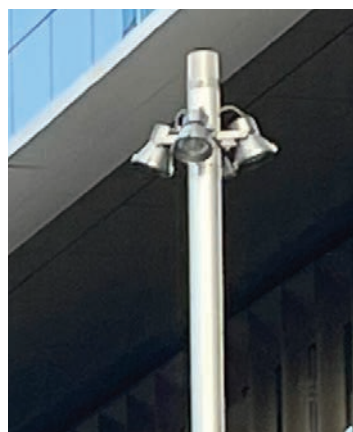
Multi-head, directional luminaires
