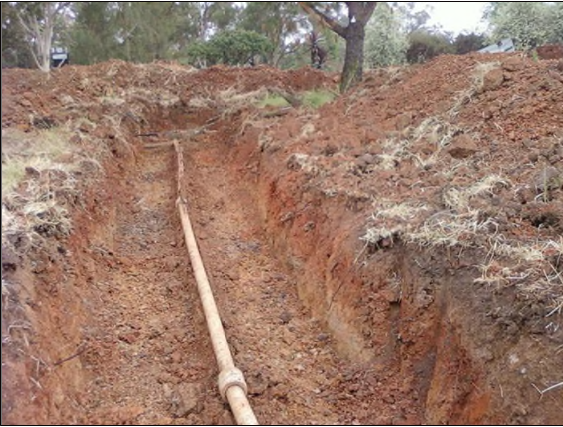
Image 1 Example of Bonded (non-friable) Asbestos Containing Pipe
