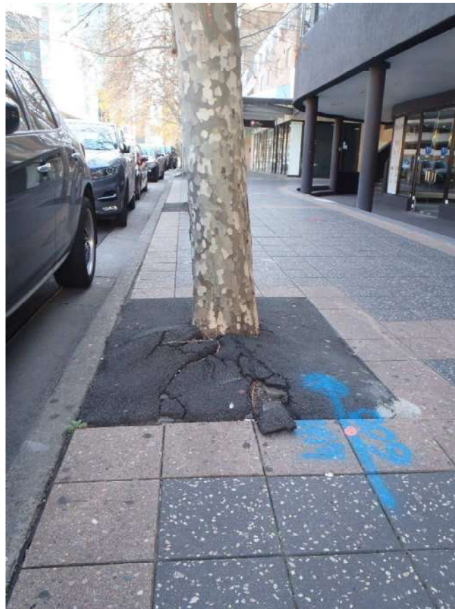
Figure 24. Photos showing T12 and T13 proposed for retention. Photo at the bottom shows displacement of asphalt indicating root zone upheaval indicating inadequate soil volume. Date: 8 August, 2023. Source: ELKE
