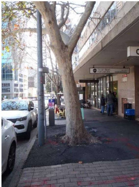
Figure 11 View looking north to T5 with asphalt installed around the tree base. Surface cracks and uneven ground is visible and installed services and posts (e.g. parking meter). T4 is proposed for removal. Date: 8 August, 2023. Source: ELKE
