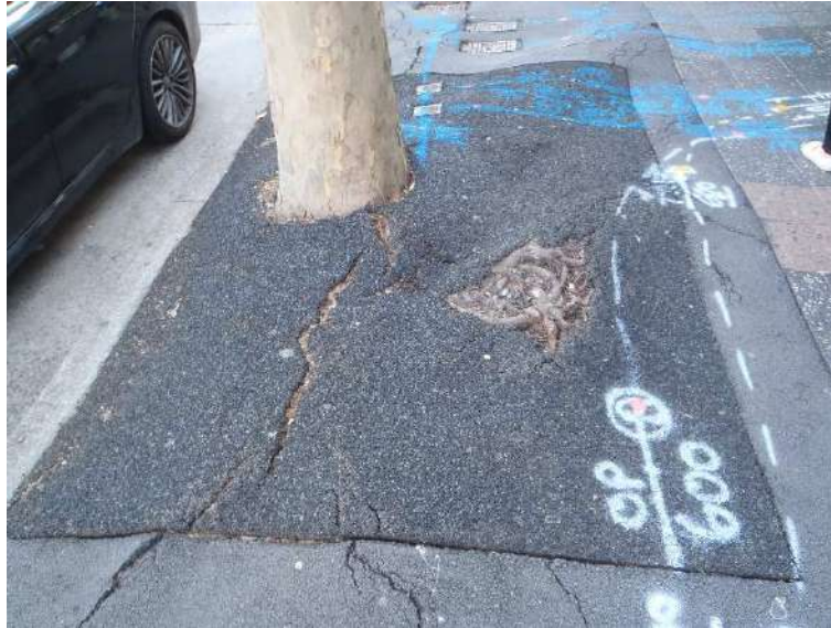
Figure 21. Photo above showing the base condition of T11 . Proposed for Removal. Surface mounding, cracking, exposed roots (asphalt cover has gone), and multiple services pits within close proximity of the tree (top of photo) and survey marks showing services. Date: 8 August, 2023. Source: ELKE
