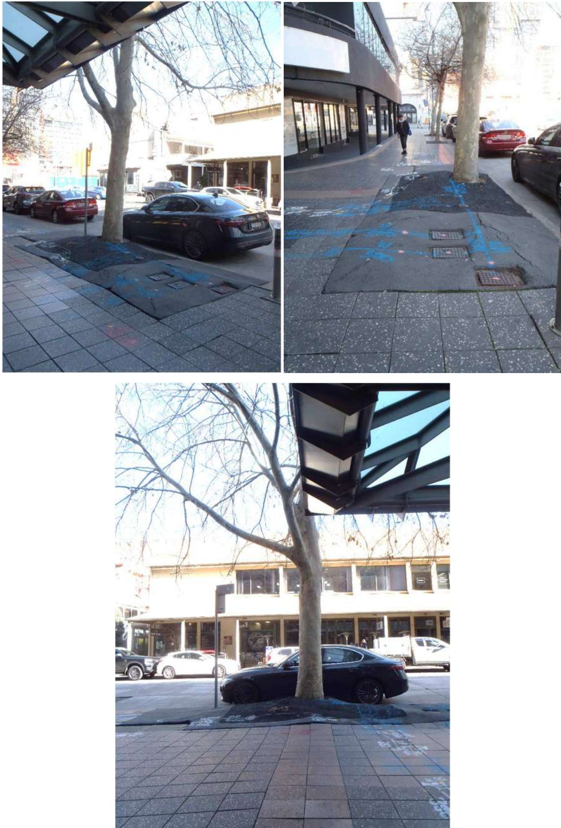
Figure 20. Photos above showing the base condition of T11 . Proposed for Removal. Surface mounding and cracking and multiple services pits within close proximity of the tree. Date: 8 August, 2023. Source: ELKE
