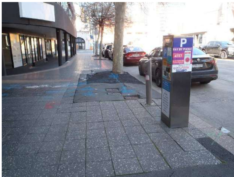
Figure 19. View looking south showing the base condition of T11 . Proposed for Removal. Surface mounding and cracking and multiple services pits within close proximity of the tree. Date: 8 August, 2023. Source: ELKE
