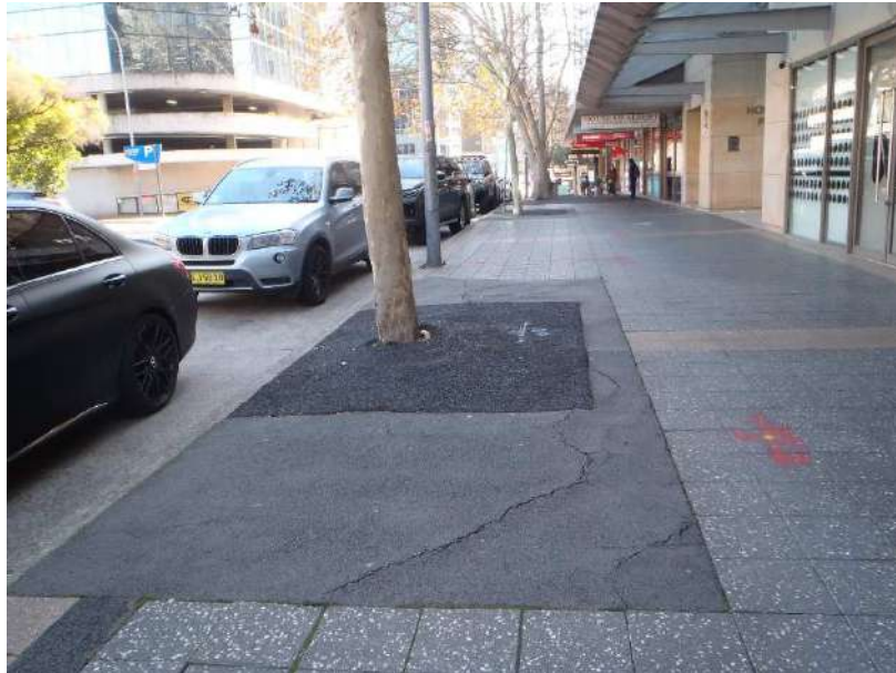
Figure 18. Base condition of T10 . Proposed for retention. Surface cracking in asphalt visible. Date: 8 August, 2023. Source: ELKE
